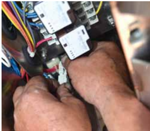
Step 14: Trim the excess power lines down and attach the connector. Then reconnect the two connectors.
