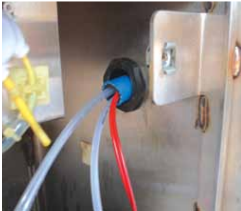
Step 11: Feed the lines through the interior lock nut and attach the lock nut to the interior of the hole.
