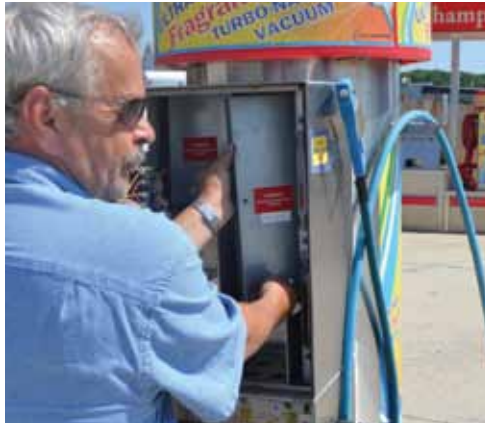
Step 3: Remove the Power Cover inside the unit.
